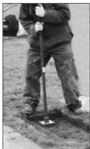
Soil should firstly be properly prepared, vigorously rammed and tamped (firmed and consolidated) with a suitable heavy metal rammer as shown on the left before the pre-cast reinforced concrete, hardstone or granite foundation slab is carefully positioned to help ensure the memorial's long term stability. Sharp sand can also be used as a fine levelling agent.
