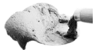
If the cement begins to dry out a little before use **do not** add additional water. By adding more water the cement's chemical reaction will be changed and the strength of the cement will be weakened.
