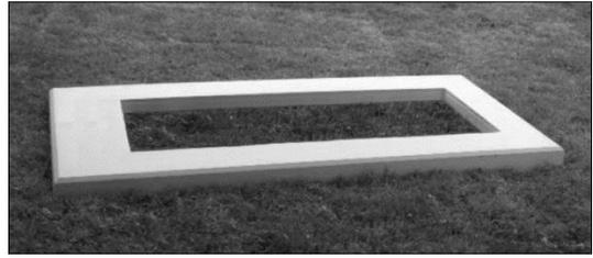
Purely as an example, and in its simplest form, a typical single width full grave memorial foundation would comprise of a reinforced concrete frame landing as shown above.
